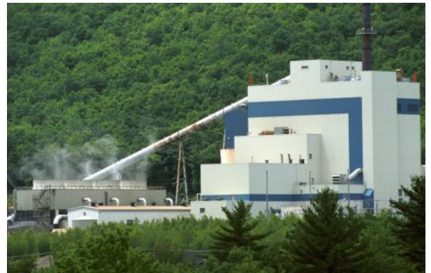
Cyrpto-mining center on-site power generation, Nesquehoning, PA: Jon Harris, The Morning Call, August 4, 2021
