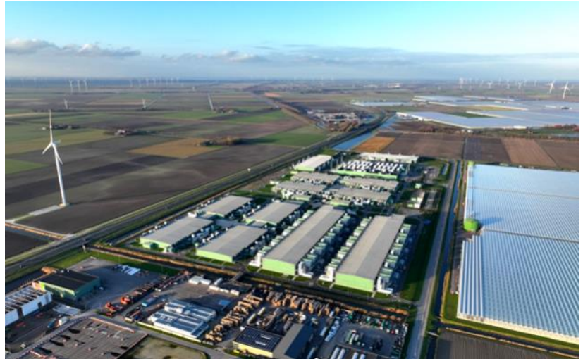
Hyperscale Data Center Example: Fleming Construction Group, 2025
