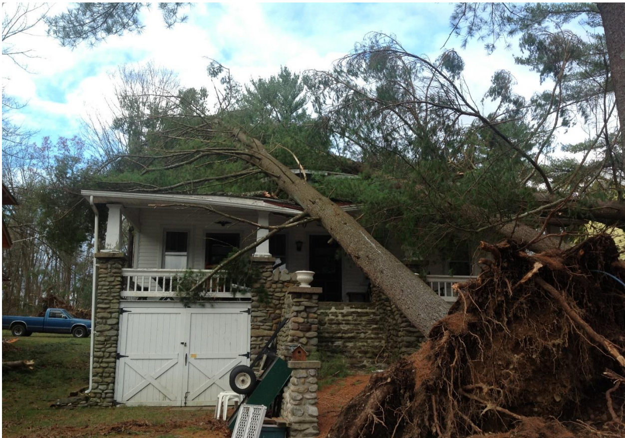
Figure 26 - Uprooted Trees Lay Atop Crushed House
