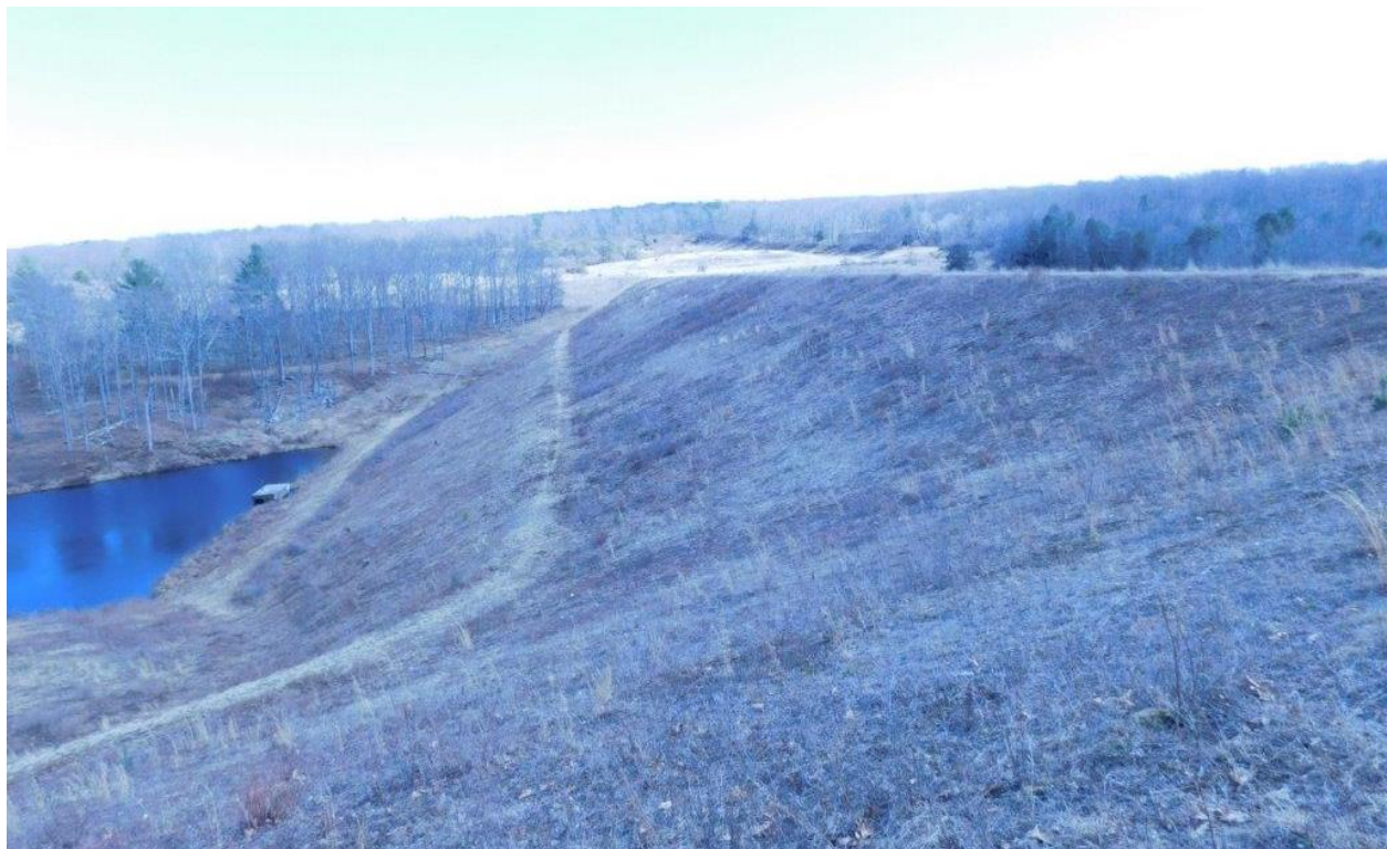
Figure 43 - Leavitt Branch Flood Control Dam
