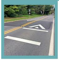
**Description:** Raised humps in the roadway, typically 3—4 inches high, intended for low volume and low speed roadways. Speed humps are most effective when placed in a series. Speed humps are the most popular traffic calming measure due to their effectiveness at reducing speeds, ease of implementation, and relatively low cost. Speed tables are speed humps with a longer flat top.
