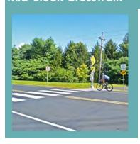
**Description:** A crosswalk that is a not located at an intersection. Additional warning devices for drivers are required to increase pedestrian safety compared to typical crosswalks at intersections. A mid-block crosswalk can include advance signage and pavement markings. Other design treatments could include a pedestrian refuge island or raised crosswalk.
