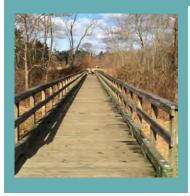
**Description:** Elevated walkway that is constructed as a series of low-height bridges through sensitive areas with seasonably variable water depths or low strength soils, such as wetlands. Boardwalks typically include a curb or handrail along at least one, often both, edges.
