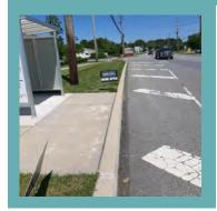
**Description:** A level loading area where the front, side, or rear door of a bus open to receive and discharge passengers. The clear area allows deployment of a front door ramp on the bus. The loading pad should be a firm and slip-resistant surface, such as concrete. Additionally, it should be free of conflicts, such as landscaping or street furniture. The loading pad should be a minimum of 5 feet wide along the curb and 8 feet deep.
