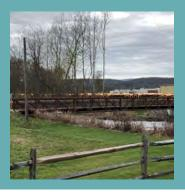
**Description:** Bridge specifically for use by pedestrians and bicyclists to cross a stream, water body, steep grade, or other existing feature. The design of the bridge should be based on anticipated users, including maintenance or emergency vehicles. Steel, fiberglass, and wood are materials typically used for pedestrian or trail bridges.
