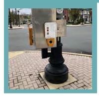
**Description:** Traffic signal equipment for pedestrians can include pedestrian pushbuttons, accessible pedestrian signals, passive detection for bicyclists or pedestrians, pedestrian signal heads, and pedestrian countdown signal heads. Accessible pedestrian signals (APS) communicate information about the WALK and DON'T WALK intervals for pedestrians who are blind or have low vision. Countdown pedestrian signal heads show how much time remains before the traffic signal changes.
