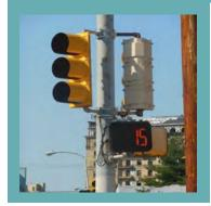
**Description:** Signal timings for pedestrians can include a leading pedestrian interval, which gives pedestrians a head start when entering an intersection. This enables pedestrians to establish their presence and enhances pedestrian visibility.
