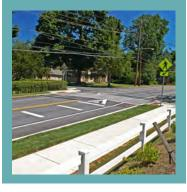
**Description:** Marked and elevated areas that are an extension of the sidewalk at mid-block locations or intersections. They can be used to increase pedestrian safety, calm traffic, and add to the community character. When used for traffic calming, they are most effective when placed in series. They may be constructed of asphalt, brick, or stone pavers.
