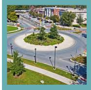
**Description:** An intersection design treatment that reduces conflict points and slows traffic. Traffic approaching the intersection yields to traffic circulating around the roundabout. Splitter islands at the entries help to slow and direct traffic and serve as pedestrian refuge areas. In some situations, roundabouts can provide increased capacity and reduced delay when compared with traffic signals.
