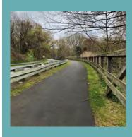
**Description:** A combined bikeway and walkway that is designed for shared use by bicyclists and pedestrians of all abilities, as well as other non-motorized modes of transportation. Trails along or adjacent to a roadway are physically separated from vehicular traffic by a verge, fencing, or other barrier.
