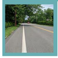
**Description:** Reduced excessive lane widths can help to slow traffic by providing a defined area for travel. Also, a reduction in lane widths can provide additional space for bicyclists and pedestrians. Lane widths can be defined by edge line striping, curbing, or other physical roadside treatments.
