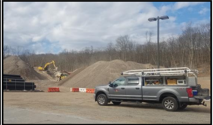
New Hotel Construction in Pocono Township
