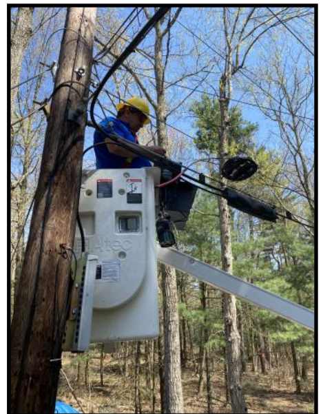
Installing Optic Fiber on Kroucher Road
