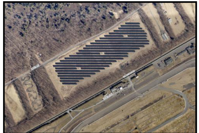
Established Solar Field at Pocono Raceway
